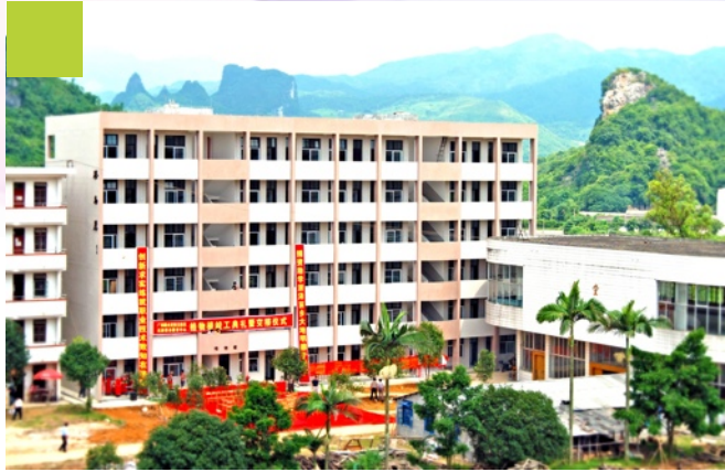
Engineering students contributed to the structural design and construction of a school and dormitory in Guangxi (Ge Wu Lou Project)
